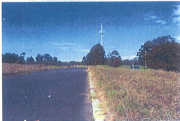
Photograph looking South along Western boundary of subject site. Note: Telecommunications Tower in the distance.
