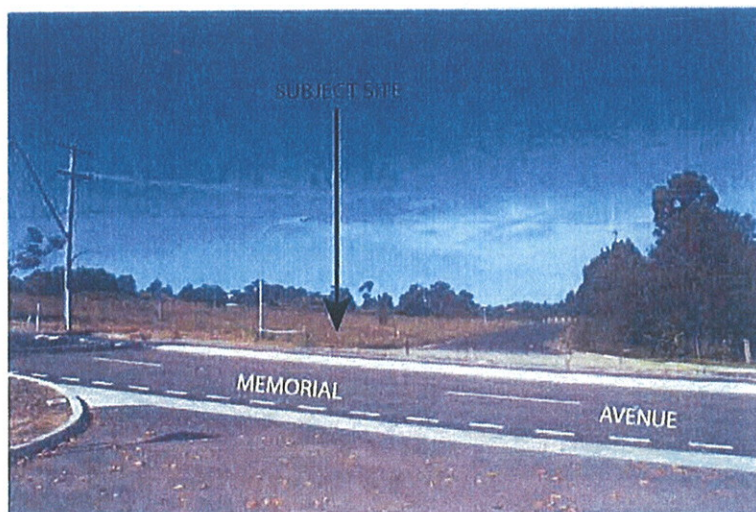
Photograph showing subject site viewed from northern side of Memorial Avenue
